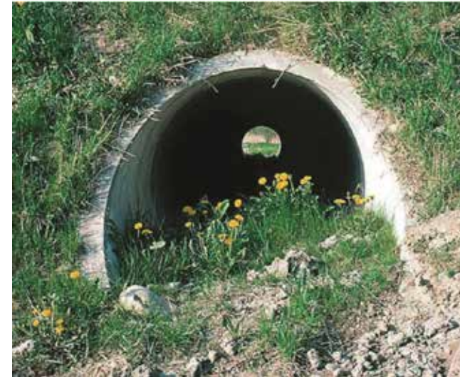
Culverts for movement of water and wildlife
